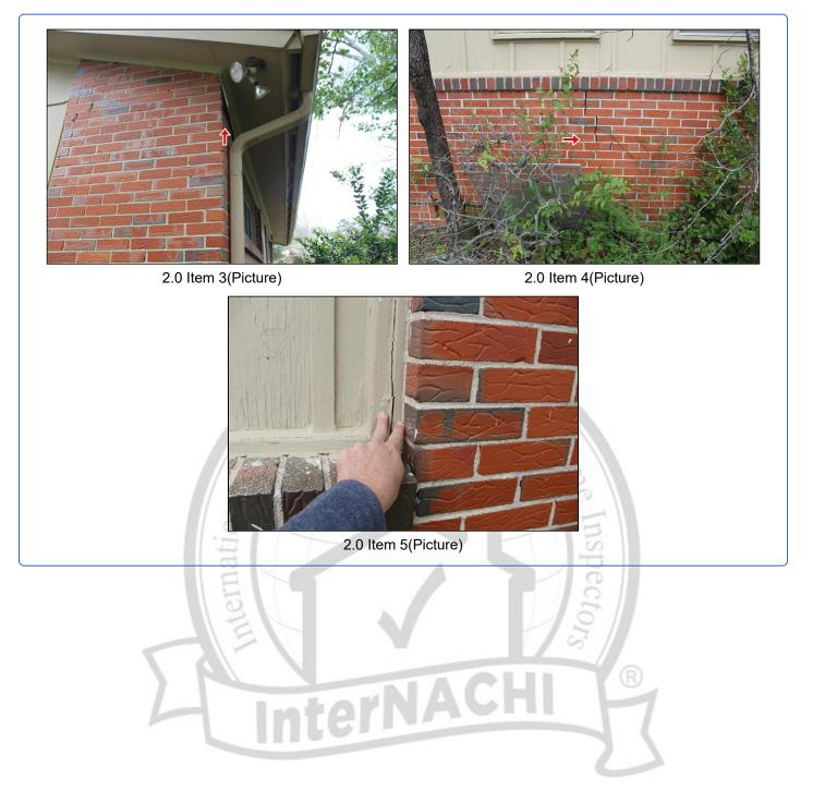
• Areas of bare wood / peeling paint need to be scrapped to remove loose paint, primed, caulked and painted at the exterior.
